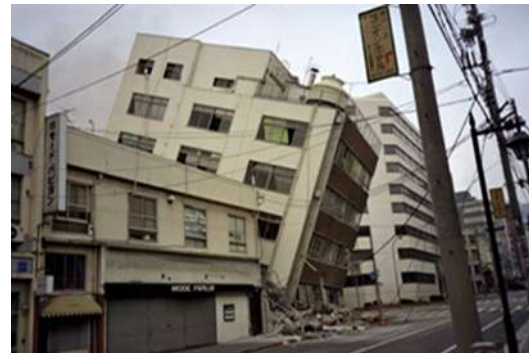
Fig.1 Deterioration of Fifth Storey of a Building in the Kobe Earthquake, Japan, 1995 (Source- Poncet L. and Tremblay R., 2004)
